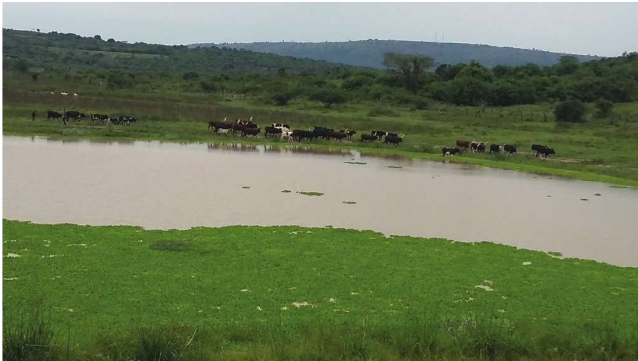
Plate 2: Makukulu valley dam in Kaliiro Sub-county
