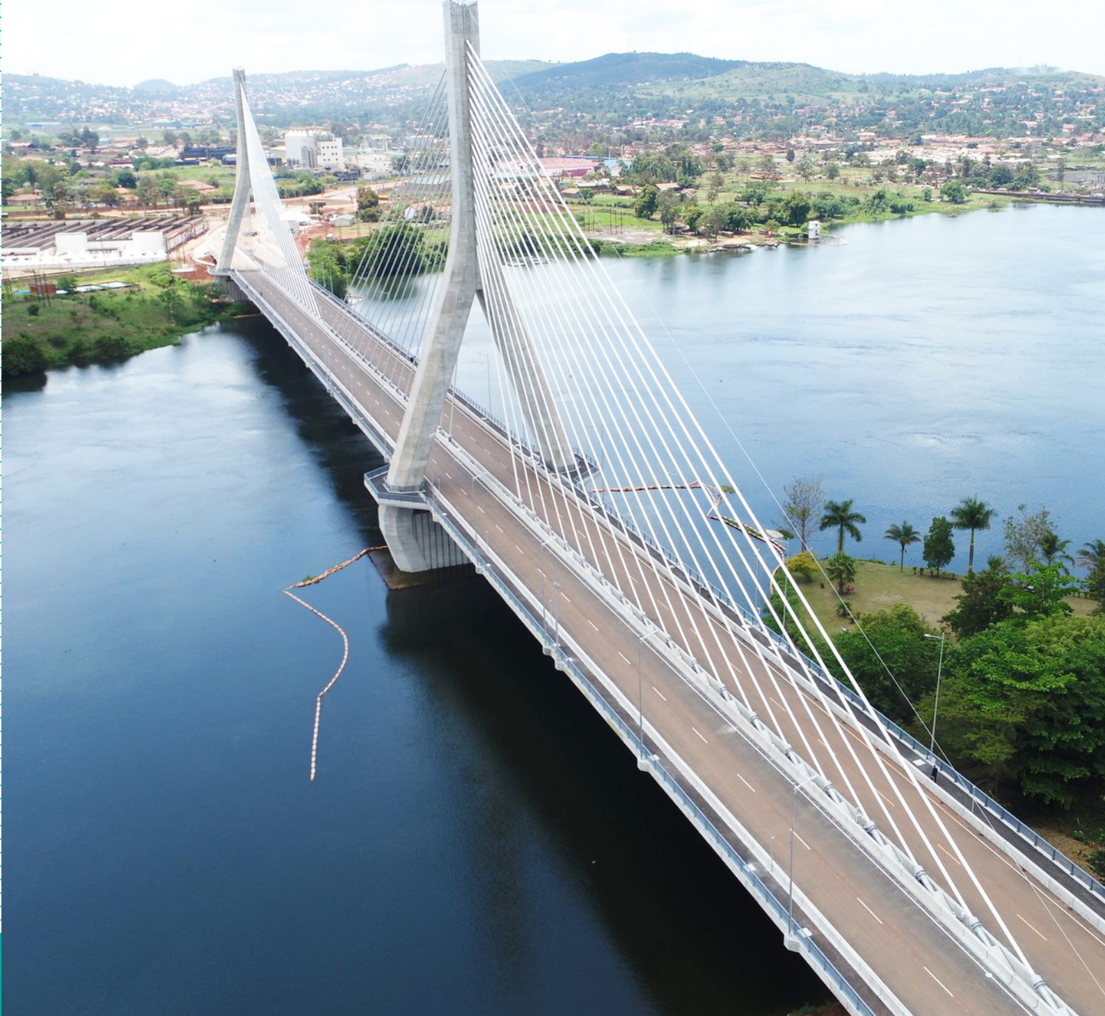
Source of the Nile Bridge
