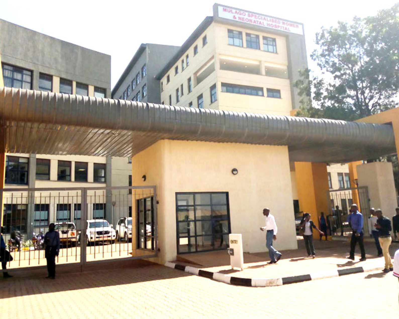
The Newly constructed Mulago Specialized Women and Neonatal Hospital Kampala
